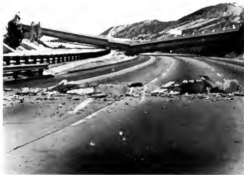
Photo 12. View north showing principal break of Reservoir segment of San Fernando fault zone where it cuts across the San Diego Freeway about 300 feet south of collapsed southeast-bound bypass bridge of Golden State Freeway. Broken pavement here was repaired soon after photograph was taken on morning of earthquake and was not examined by Division of Mines and Geology. Later examination of area showed that seams in concrete drain along east side of freeway from fault break north about to site of collapsed bridge had cumulative southward compression of approximately 8 inches (20 cm). Photo courtesy of the California Division of Highways.
